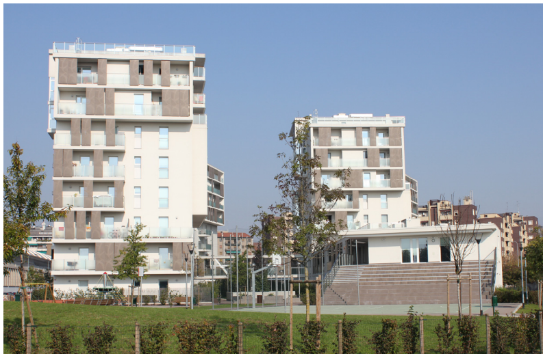
Tower building A and D
