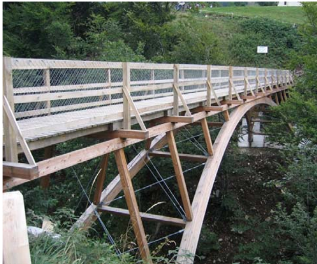
View after completion 2005
