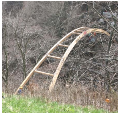
Assembly of the main supporting structure
