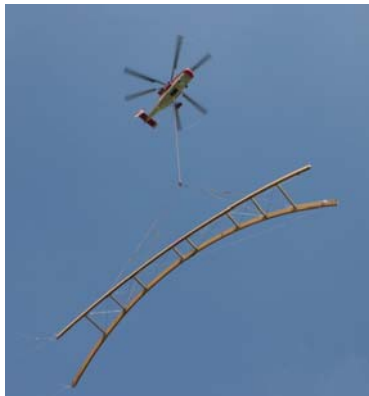
Transport of the main supporting structure
