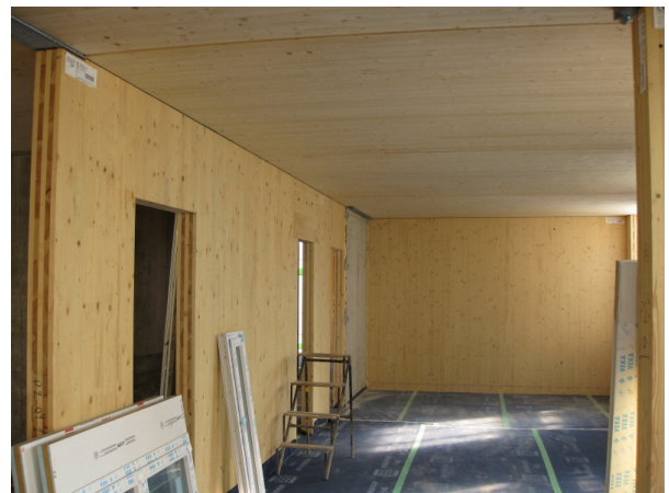
Shell construction - interior
