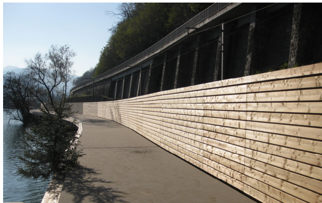
View during shell construction
