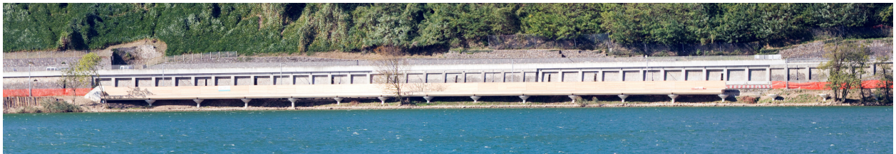
Overall view of a part of the bridge
